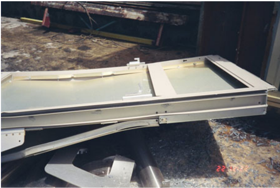
Diagnostic investigation revealed that some hooks failed while others did not.
